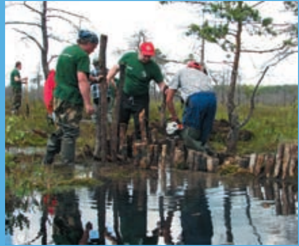
With Company help, volunteers built 34 new dams to help raise the bog's water level
