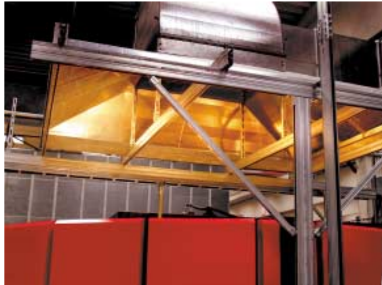
Warm air being collected for alternative use, one way of increasing plant efficiency
